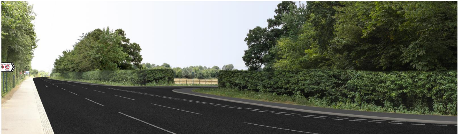
Visualisation at Year 15 (post construction) of the proposed Cantley Lane Link Road junction with the B1172 Norwich Road
